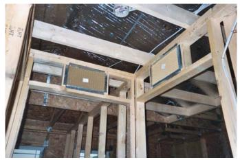
R.A.P. Transfer Grilles with baffles exposed
