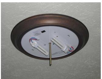
Typical for 2 Secondary Bedrooms (2) 26 Watt Pin-Type CFLs
