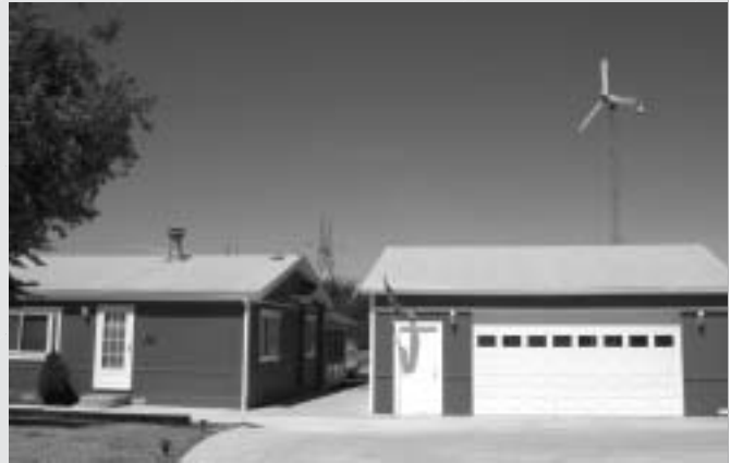
Photo courtesy Bergey Windpower
