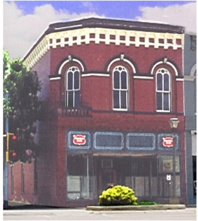
The Bishoff Hardware Building was constructed in the late 1870s. After being vacant for nearly five years, a oriental restaurant was opened in this renovated building in the Nebraska City Historic District.
