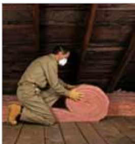
A contractor installs insulation during weatherization work.
