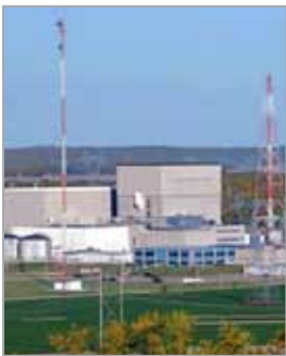
Cooper Nuclear Station near Brownville
