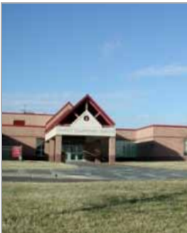
Cavett Elementary School in Lincoln uses geothermal heat pumps
